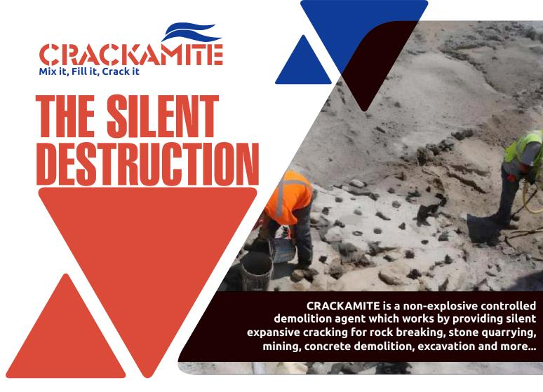
For Demolishing work in construction in tight quarters, the use of explosive agents is very restricted due to safety and environmental issues. A unique product like **Crackamite** comes as the ultimate solution. Marble, granite, limestone, plain concrete, reinforced concrete, boulders, ledge, are fractured overnight without noise, vibration or flying debris.
